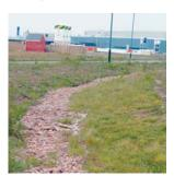
A three metre deep stone-filled vent trench was installed on the landfill side of the feeder road.
